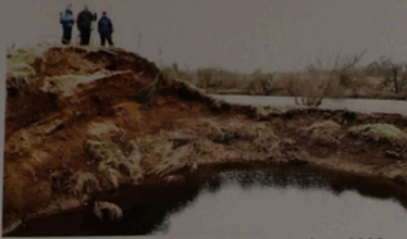
Flood embankment breach on River Isla in 2023.
